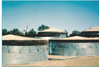
**Figura 8. Tanques desmontables OXFAM [21]**
